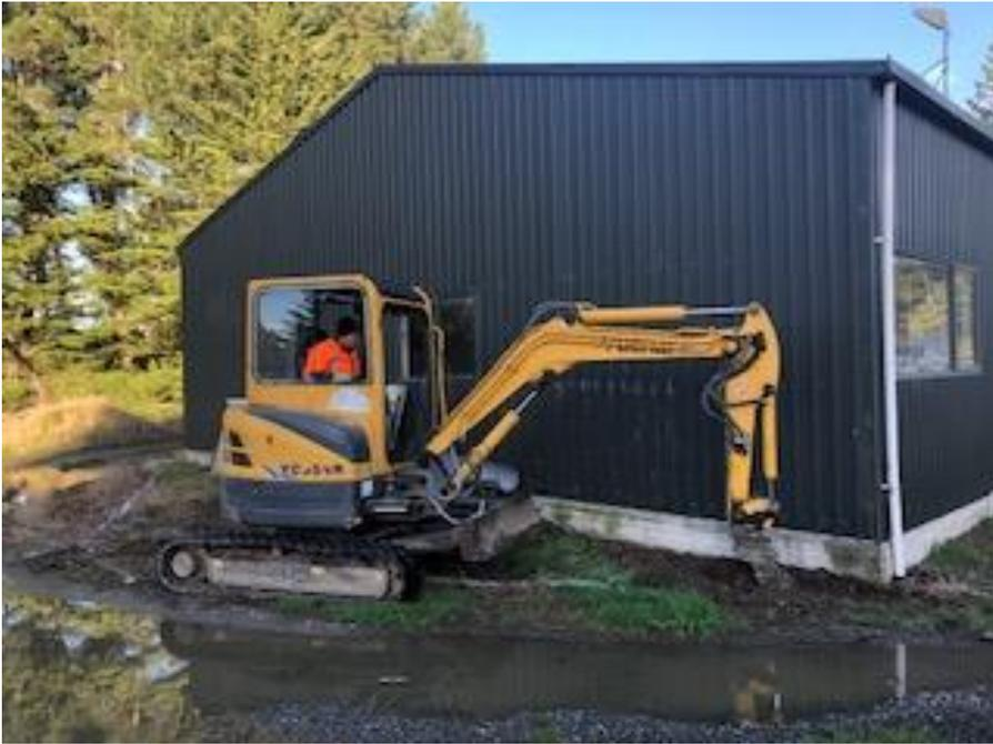
While Brian played on the digger.....(actually he was busy digging the soak pits at both ends of the shed – this will mean that all the rainwater from the shed’s roof has somewhere to go rather than pouring onto the ground besides the shed and flooding the surrounding paths and work areas each winter)
